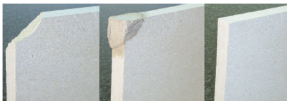
Before Applied Last Patch Limestone After
